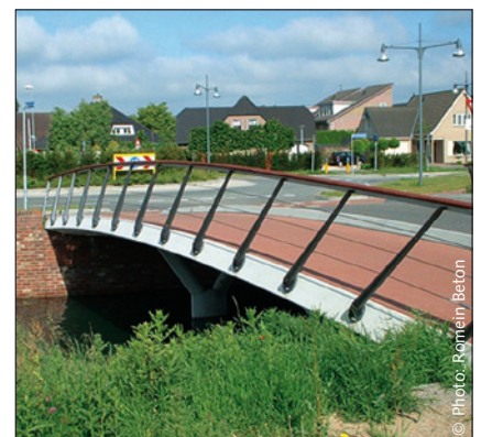
Fixing of bridge railings
