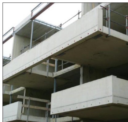
Fixing of balcony railing
