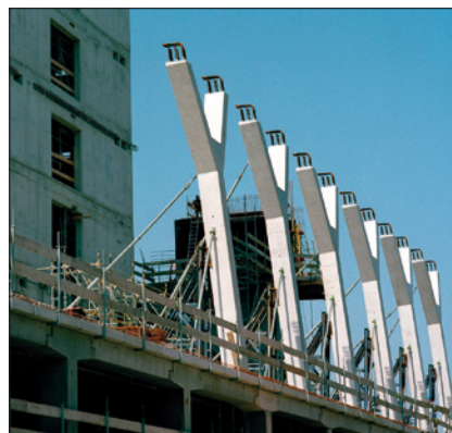
Fixing and adjusting precast elements
